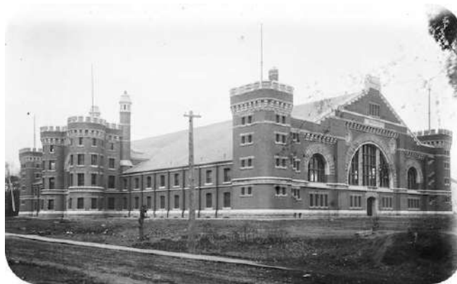
University Avenue Armouries (looking southeast)
